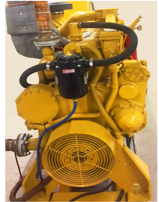
The Maxwell GSS cranked the 350 KW Caterpillar diesel generator in 1.5 seconds, compared with a 2 to 3 second start with lead-acid batteries.
