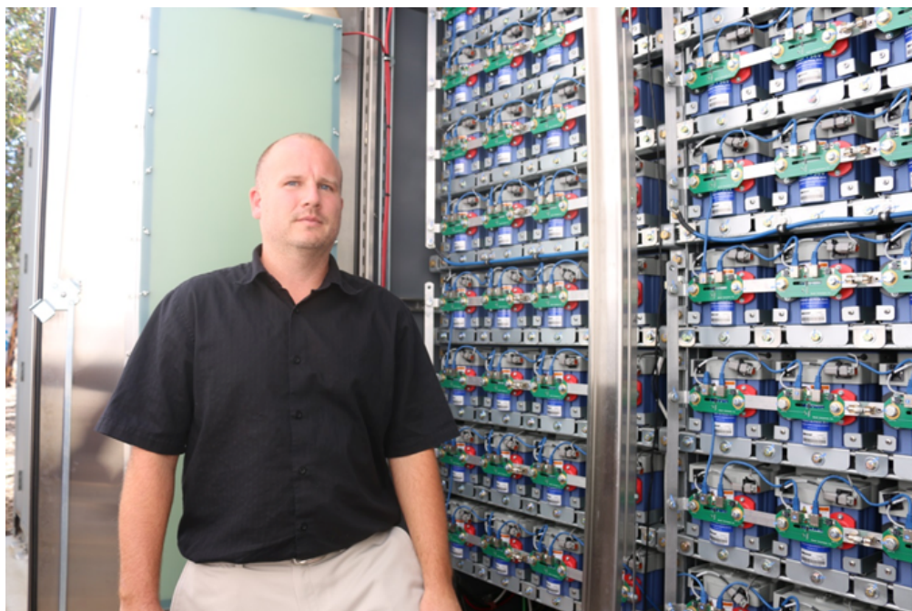
Senior Systems Engineer Mike Wilk at the site of Maxwell Technologies' ultracapacitor energy storage system, installed as part of UC San Diego's microgrid.
